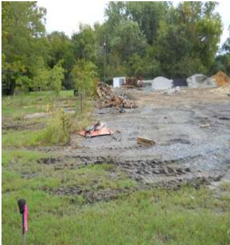
Pre- construction Gravel Run on left
