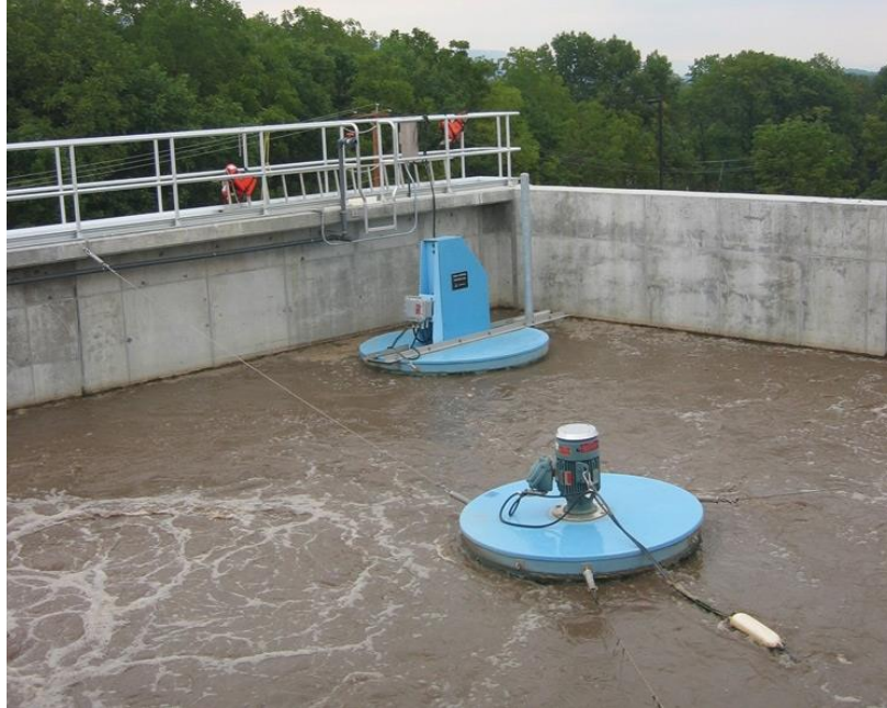
Figure 4.21: SBR Tank w/Surface Mixer/Aerator and Decant Device (Credit: Aqua-Aerobic Systems, Inc.)
