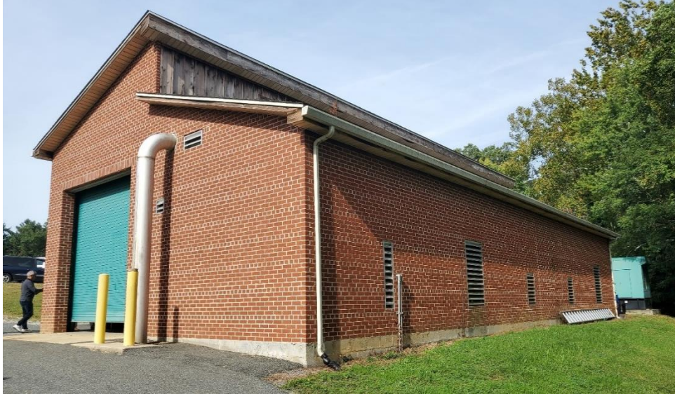
Figure 6.5: Existing Filter and Blower Building
