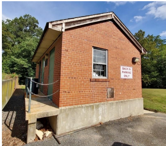
Figure 6.6: Existing Control Building
